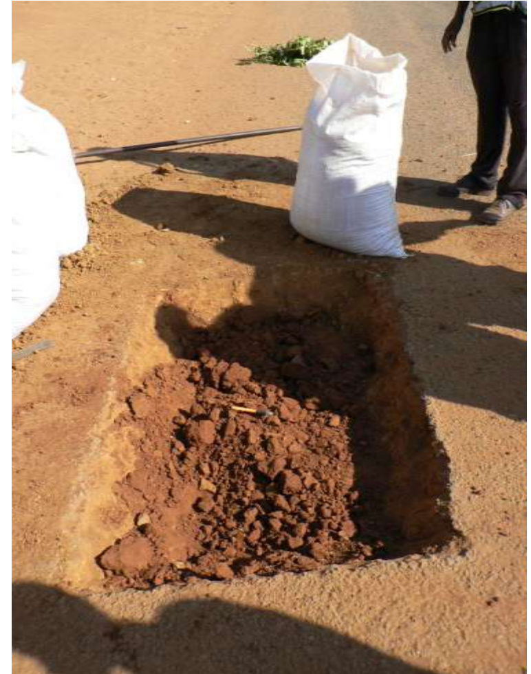
Sampling of base course material
