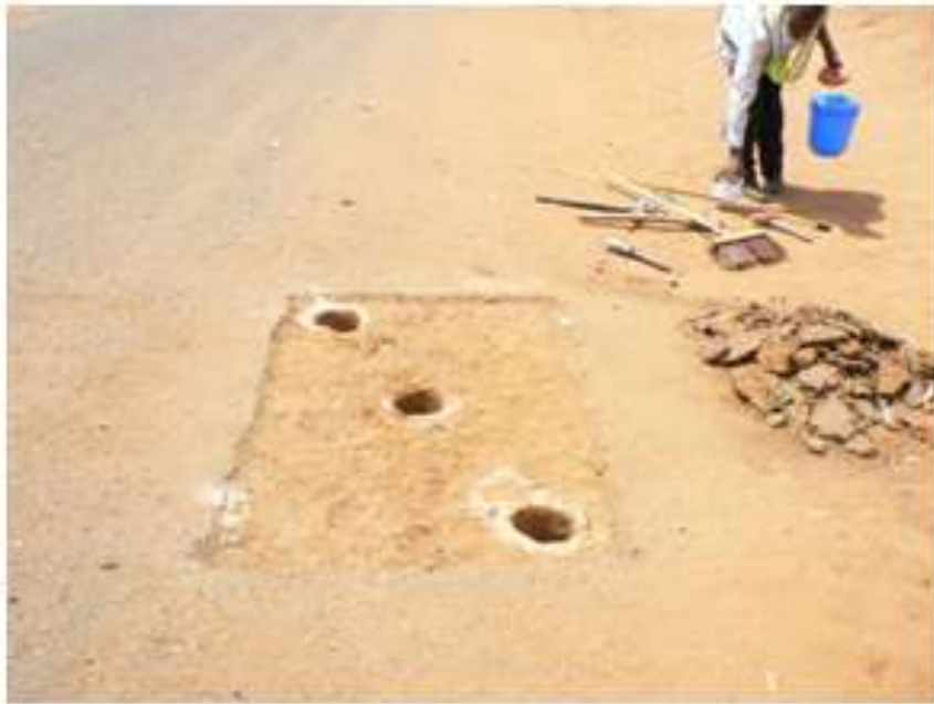
IDD testing by sand replacement method
