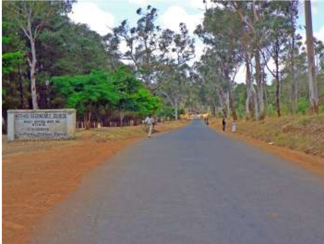
Photo: Ntchisi road (school) - constructed in 2002 Condition: Good/sound
