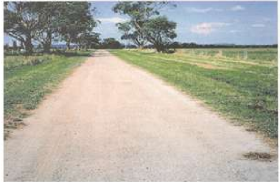
Engineered Natural Surface (ENS)
